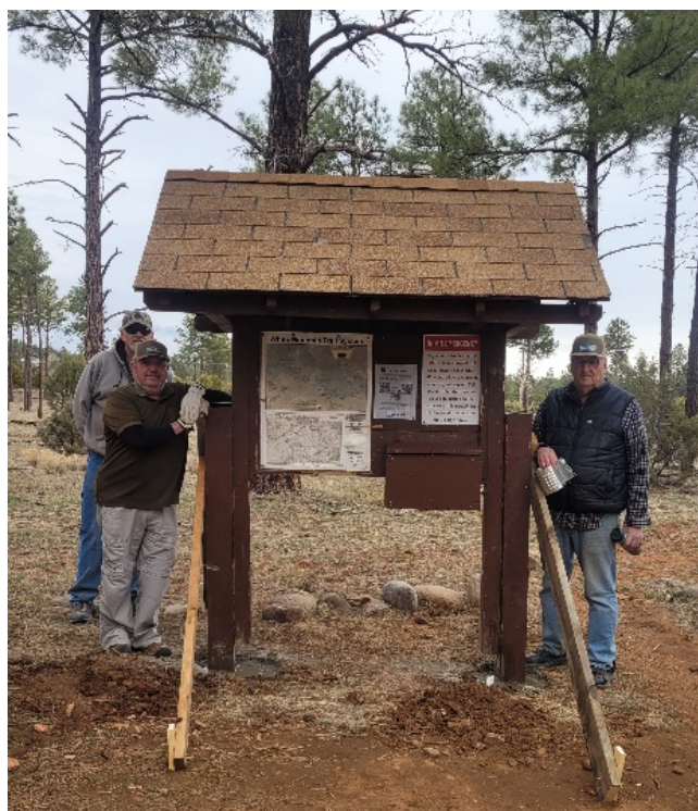
Devoted Trail Crew, repairing a kiosk this past March.
